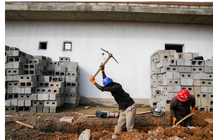
Figure 5b: Digging trenching for underground MGPS
