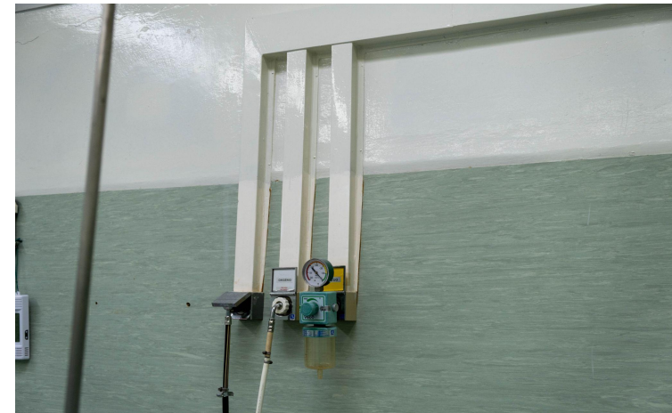
Figure 3b: Wall-mounted oxygen outlet (supplied by cylinder manifold or MGPS direct from the oxygen plant)
