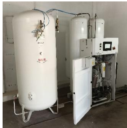
Figure 2: VPSA Plant
