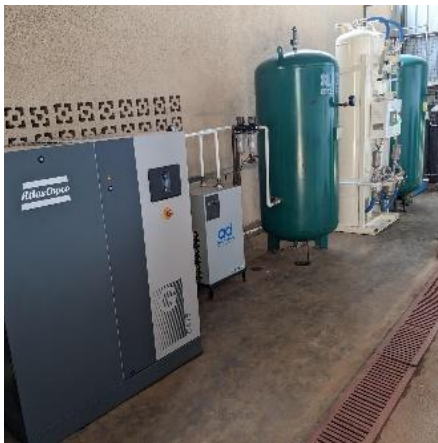
Figure 1: PSA Plant
