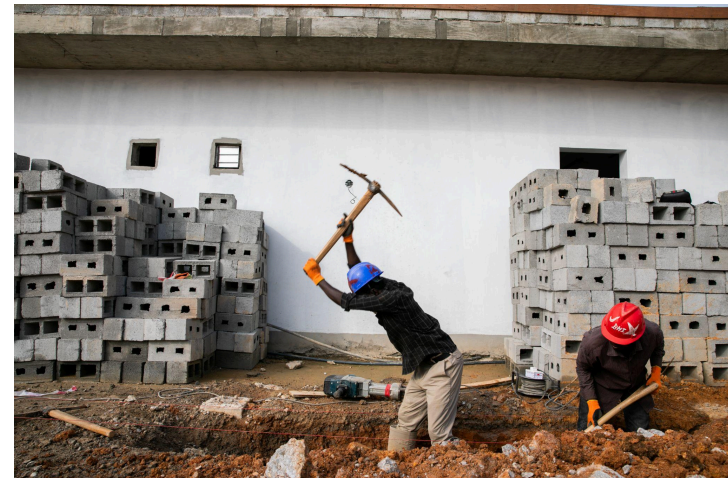
Figure 5b: Digging trenching for underground MGPS
