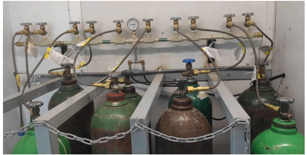
Figure 4b: Example of cylinder racking, the safest method of cylinder storage
